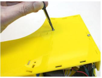
Work your way from bottom to top, aligning the tabs closest to each hole and then inserting a screw.
